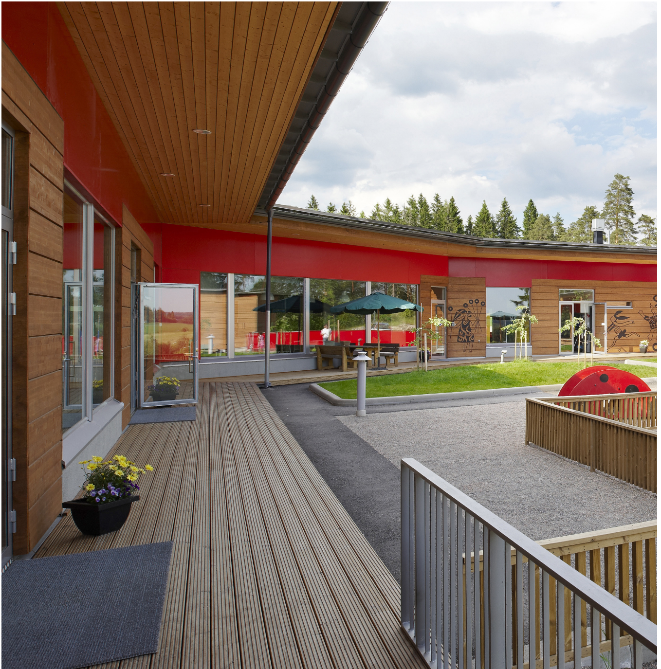
Figure 8.1. Roof overhang protects the building against weather exposure and solar radiation, Kindergarten Vekara, Pukkila, Finland.
