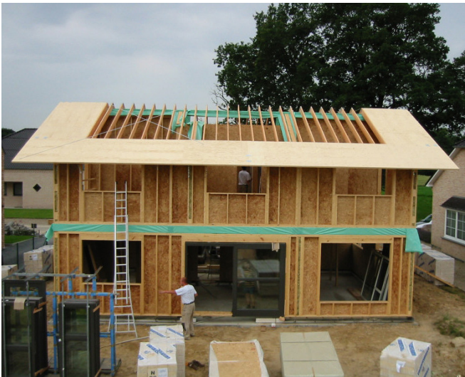
Figure 2.47. Eaves and roof overhangs from LVL-C panels.
