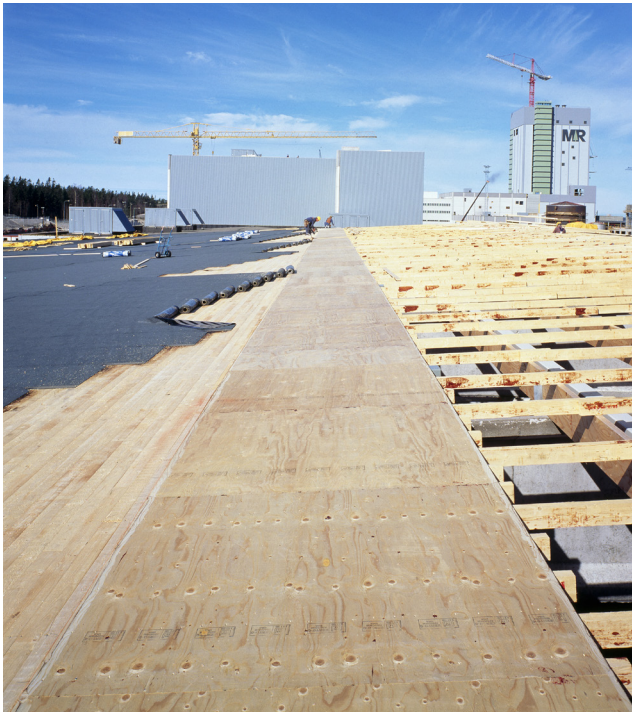
Figure 1.4. LVL-C roof panels.
