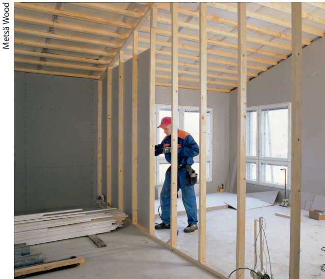
Figure 2.56. Installation of plasterboards to LVL-P wall studs.
