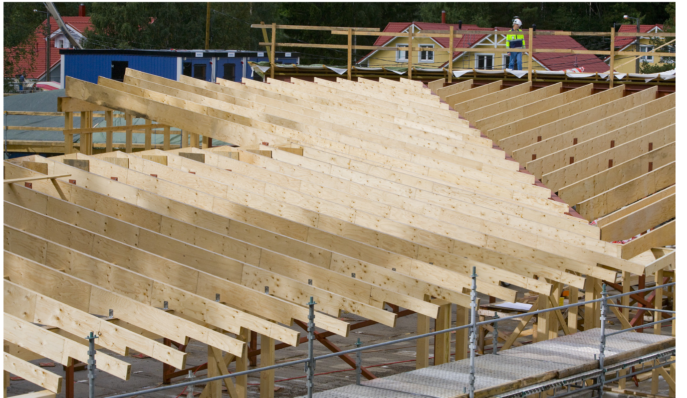
Figure 2.27. LVL-P rafters in a mono-pitch roof structure.
