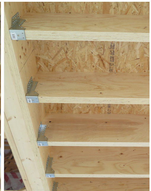
Figure 2.3. Joist hanger connections of floor joists.
