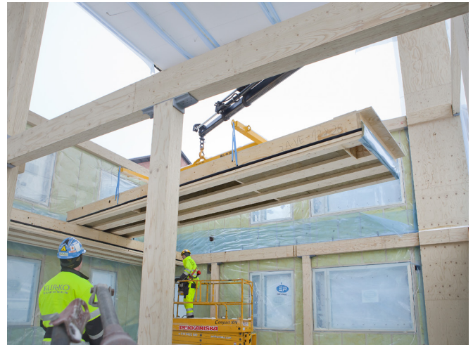
Figure 2.21. Installation of an LVL open box slab element.
