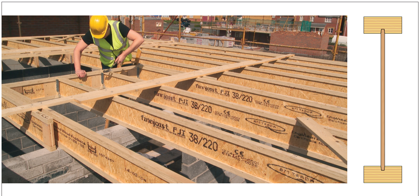
Figure 2.94. Wooden I-joist with LVL flanges.
