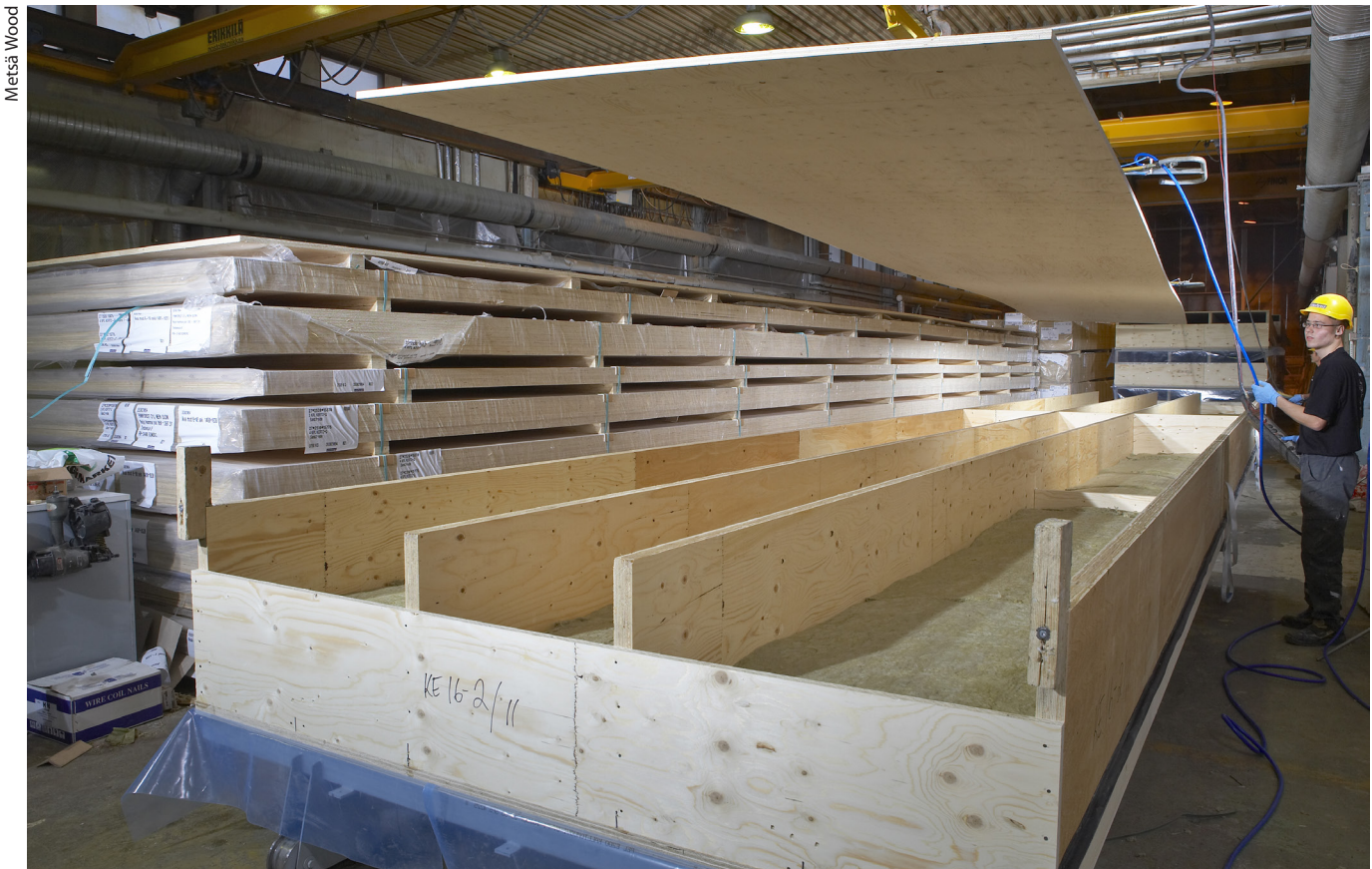
Figure 1.57: Manufacture of structurally glued LVL roof elements.
