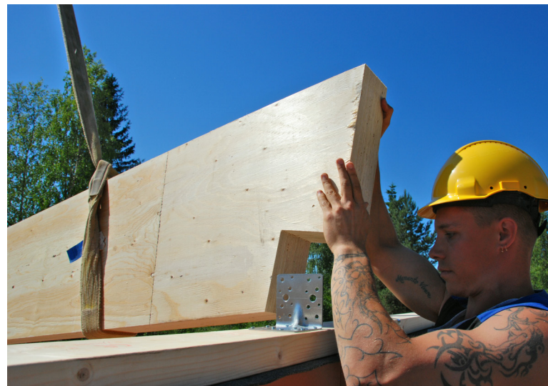
Figure 4.19. Installation of notched rafter beam.
