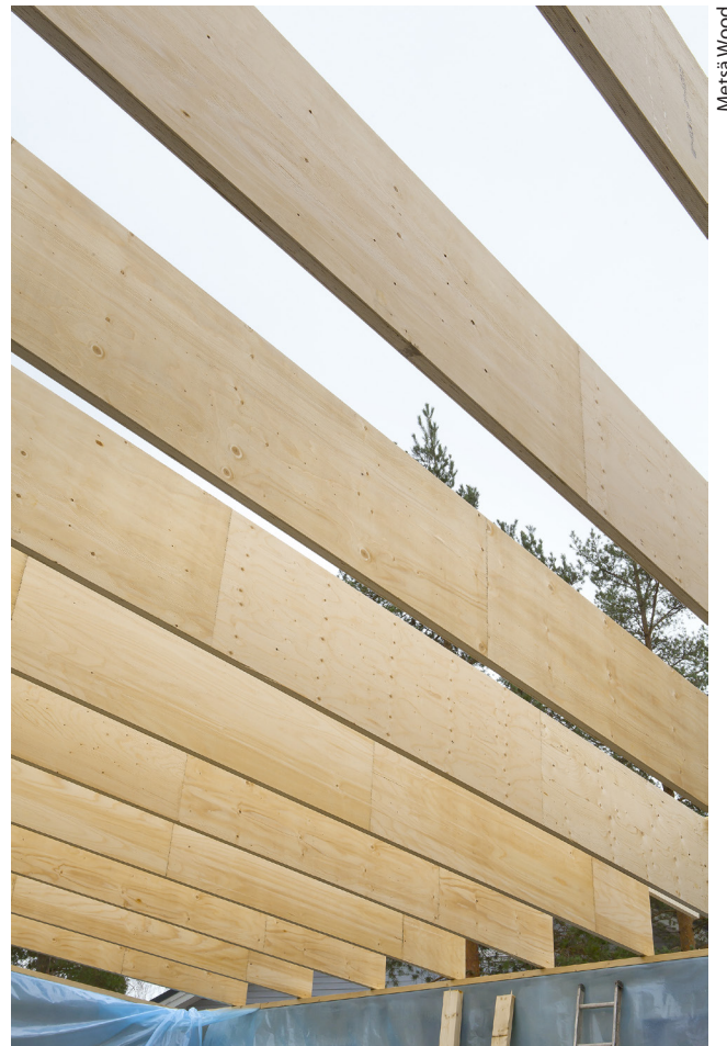
Figure 1.2. LVL roof rafters.
