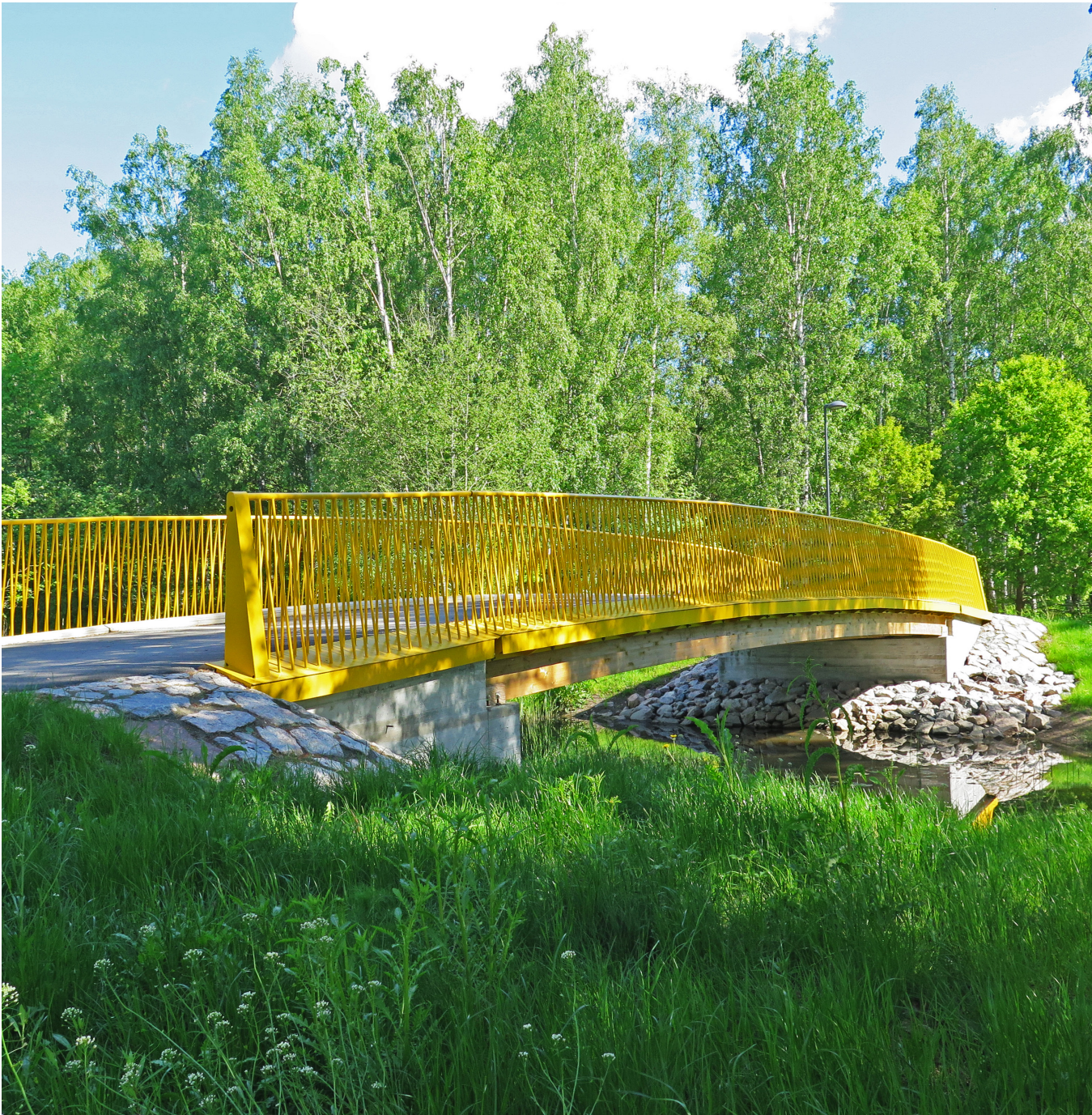
Figure 7.1. Wooden pedestrian bridge, Matinpuron, Espoo, Finland.
