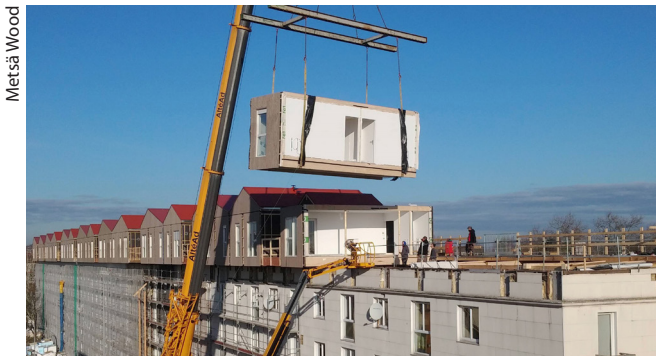
Figure 2.87. Light wooden extension floor to an existing multi-storey building from volumetric elements. Poissy, France.
