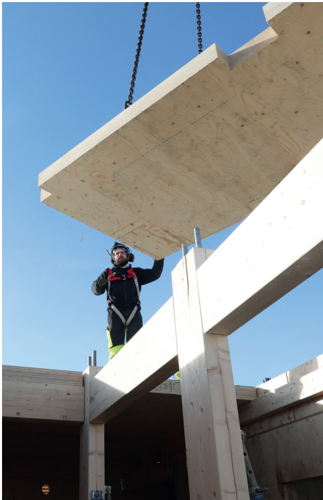
Figure 2.13. Installation of a multiple-glued GLVL-C floor element.
