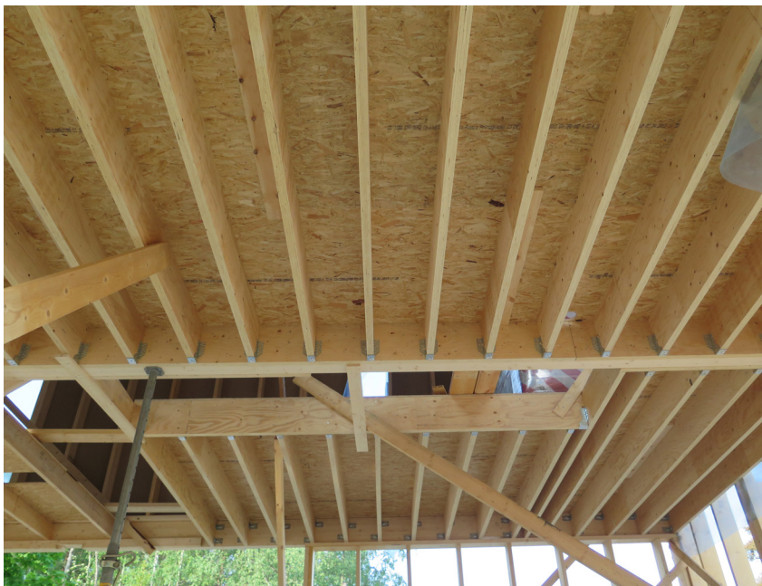
Figure 2.2. LVL-P joist floor structures.
