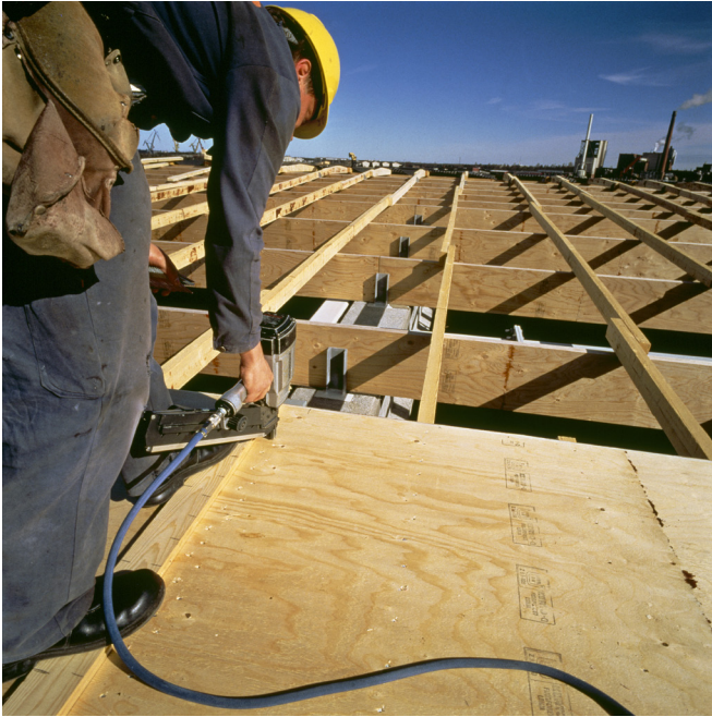
Figure 2.45. Installation of LVL-C roof panels.
