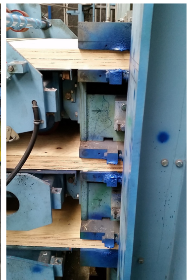
Figure 1.43. Feeding LVL billets into 3-level hot press.
