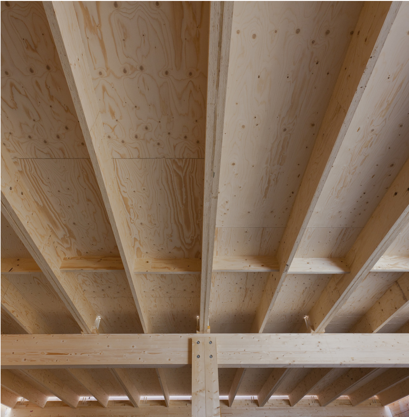
Figure 4.1. LVL roof structure, K-Rajamarket, Utsjoki, Finland.
