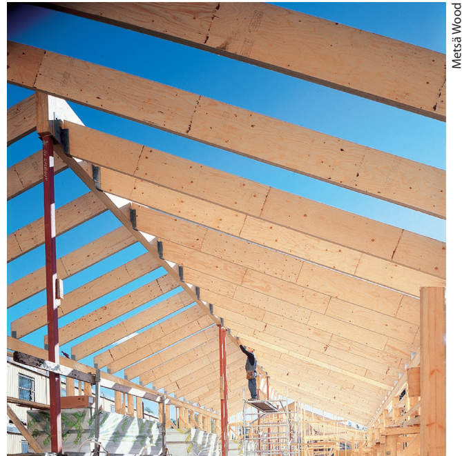
Figure 2.28. LVL-P rafters in a ridge roof structure.
