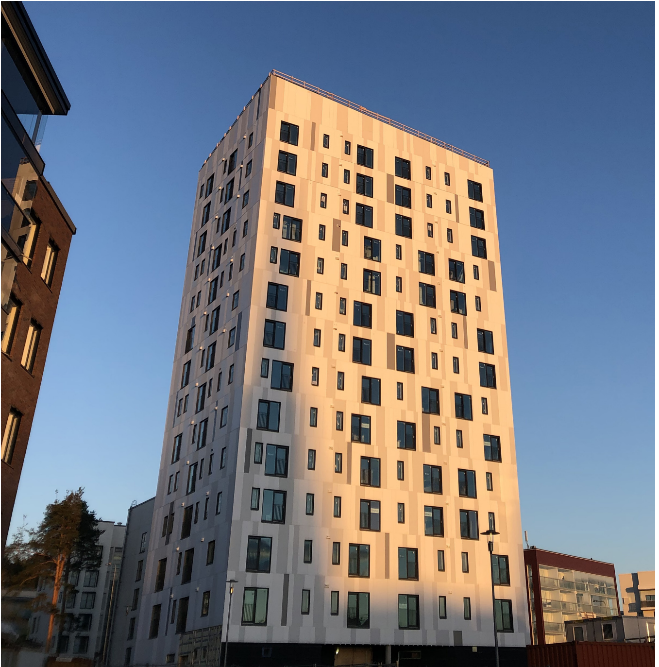
Figure 9.1. Wooden multi-storey building Lighthouse, Joensuu, Finland
