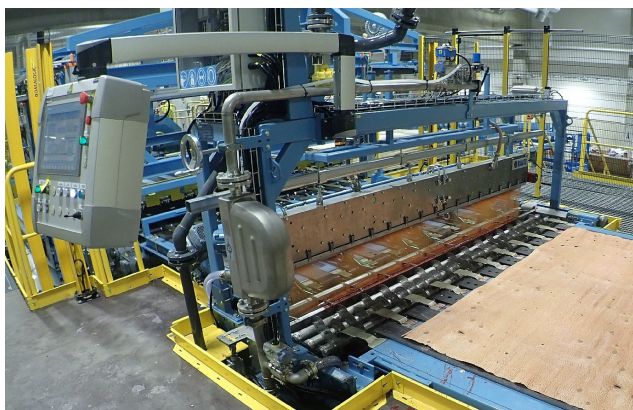
Figure1.39. Liquid extruder gluing (LEG): glue is applied to the top of the veneer as it passes on the belt conveyor.
