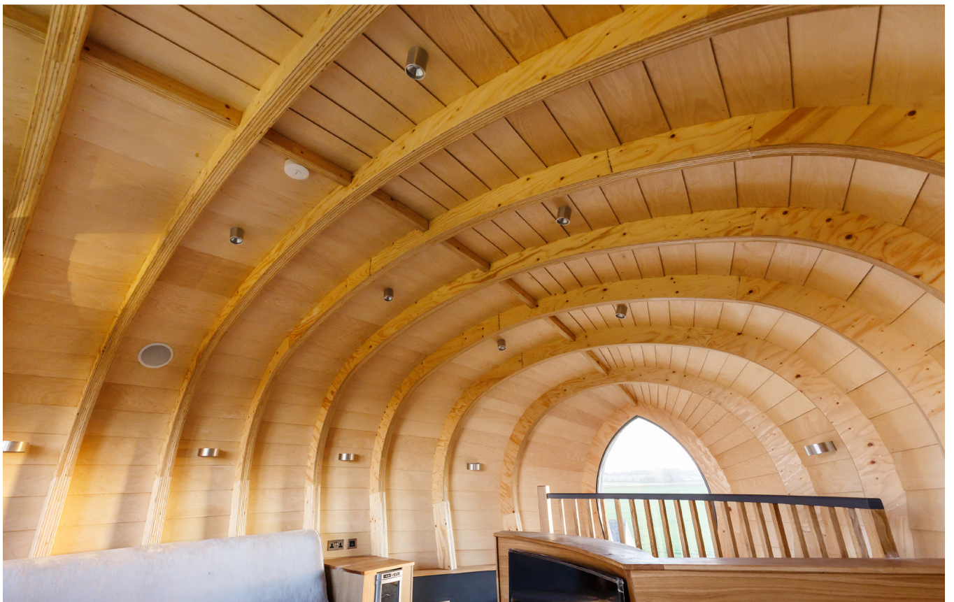
Figure 2.91. LVL-C arches for the roof structure of a windmill, UK. The structure consists of several curved members.
