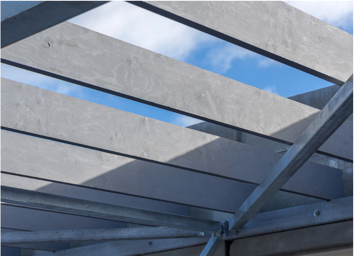
Figure 1.66. Coated surfaces of LVL beams.
